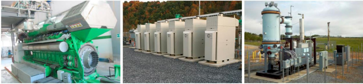
Figure 6: Electric energy production processes from landfill gas: combustion engine on the left, microturbines in the middle and gradual oxidation on the right [19]
