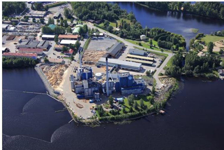
Figure 4: Aerial view of the Pursiala power plant [15]
