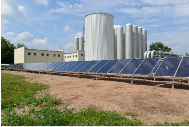
Figure 4: View of the transfer station with the south field and the two-zone storage
